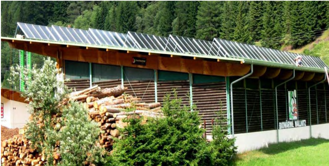
Solar district heating Solare Biowärme Mallnitz
